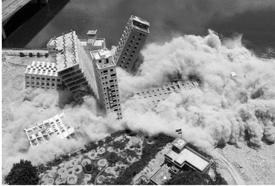
Figure 30: Blasting Demolition of Urban Village
